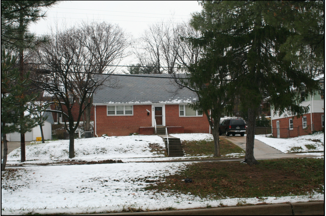
Looking east, 5909 Westbrook Drive ( EHT Traceries , 2007)
