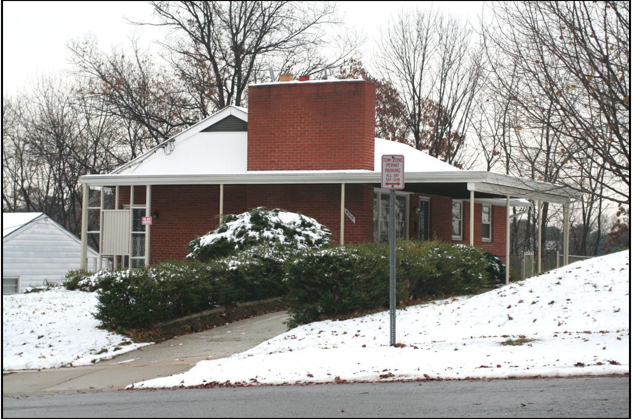
Looking southeast, 8315 Longfellow Street ( EHT Traceries , 2007)
