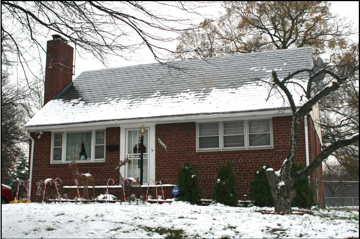
Looking southeast, 8505 Madison Street ( EHT Traceries, 2007 )
