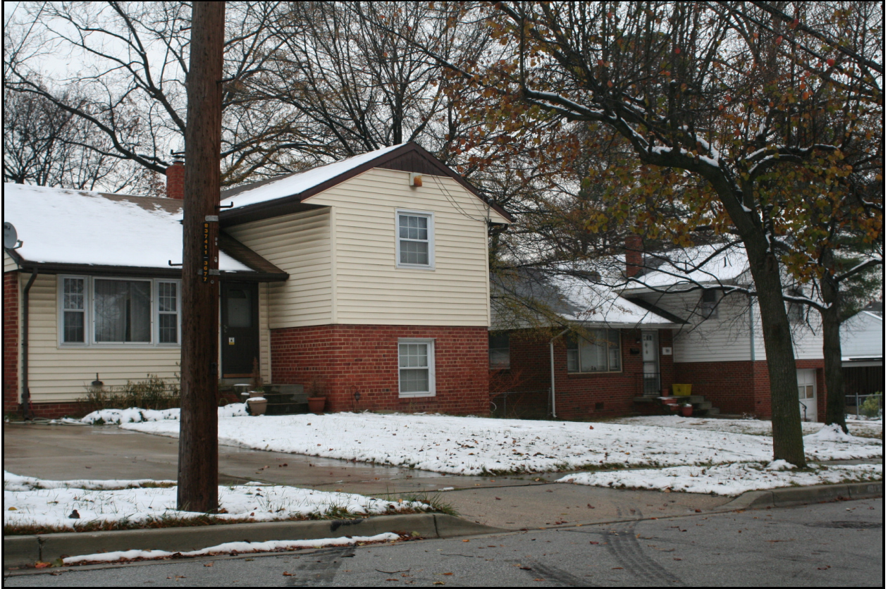
Looking southeast, 5817-5815 87th Avenue ( EHT Traceries, 2007 )
