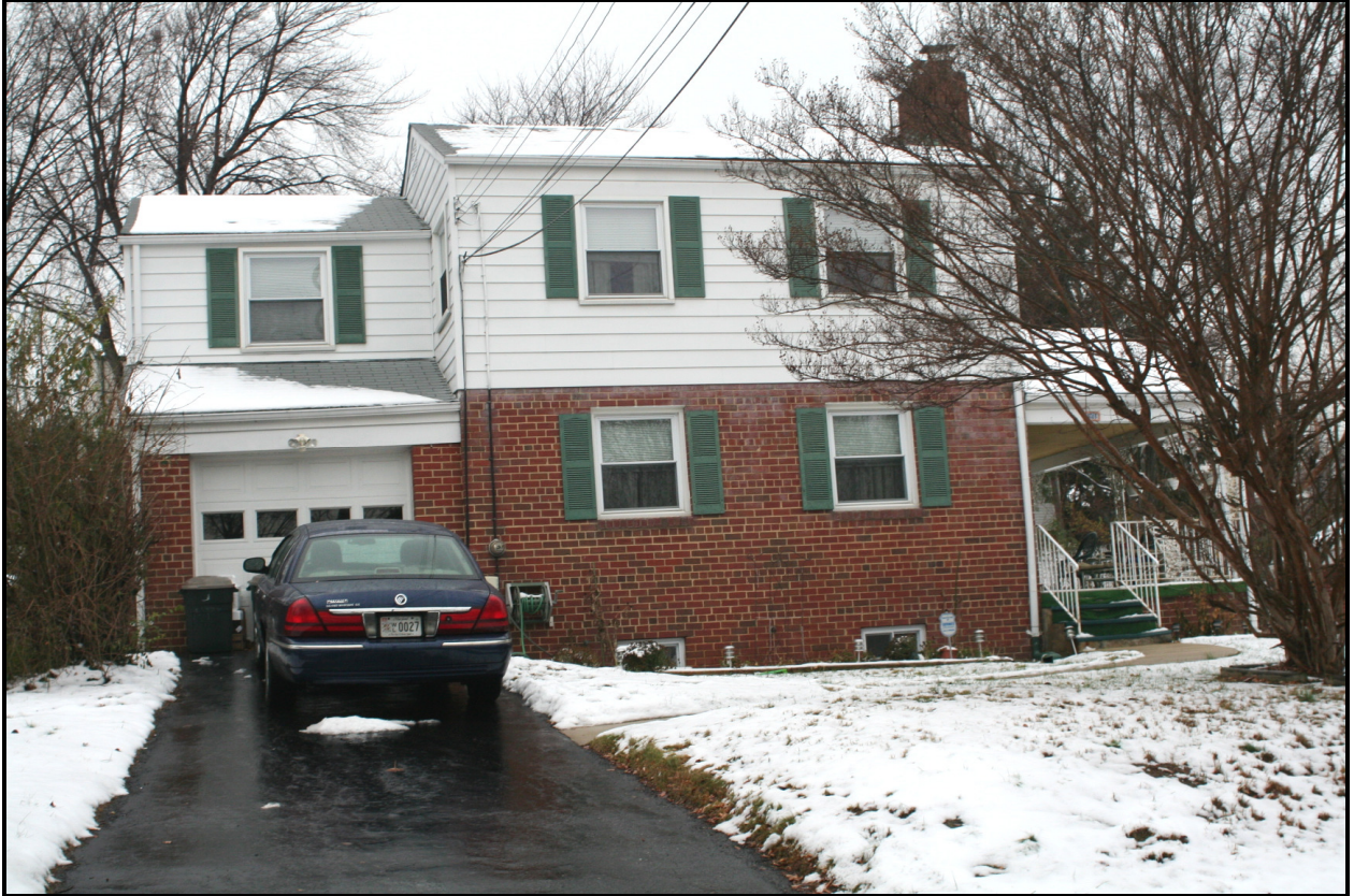
Looking west, 5708 84th Street ( EHT Traceries , 2007)
