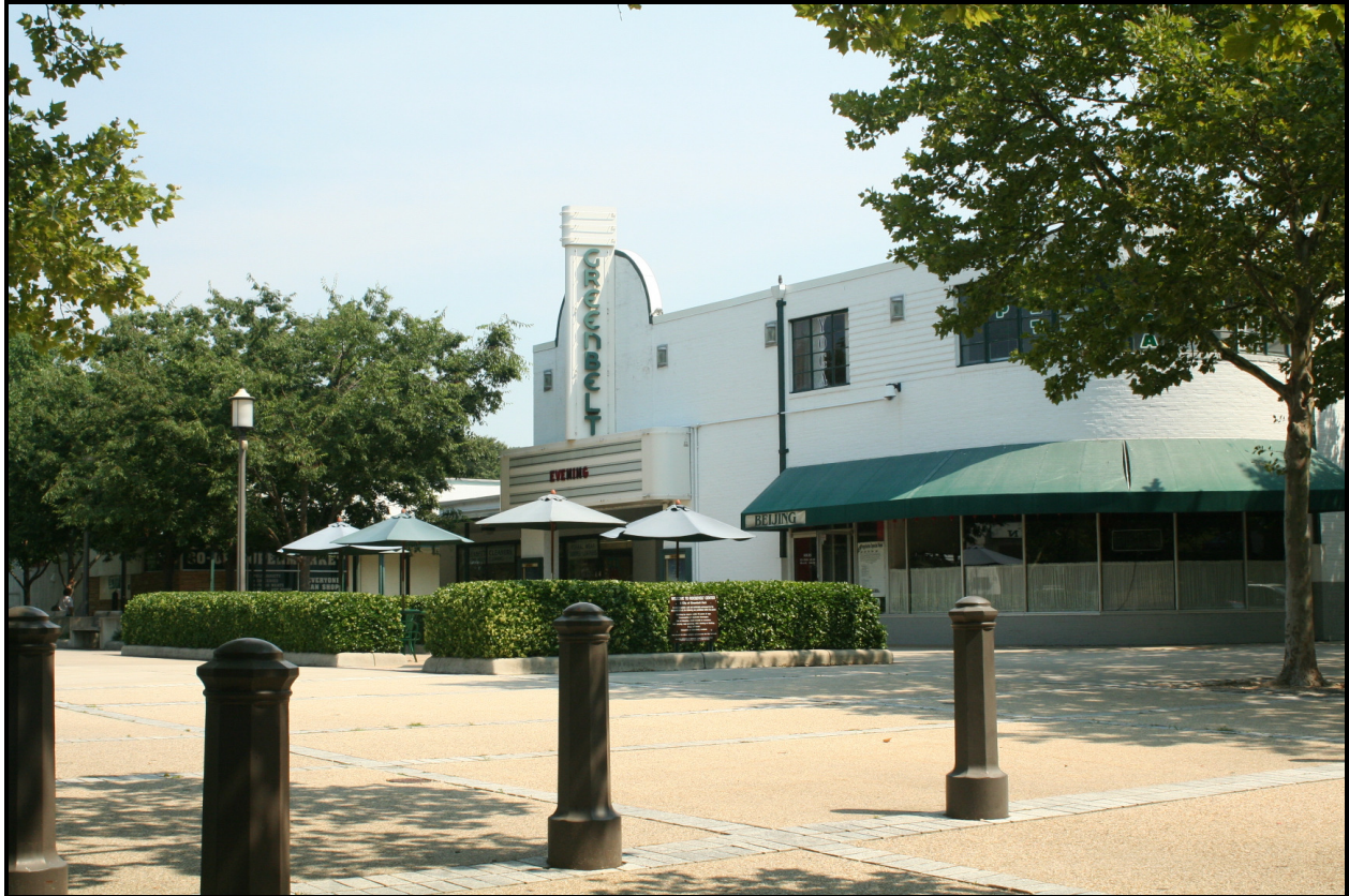
Looking north, 129 Centerway Road, Old Greenbelt Theatre at Roosevelt Center ( EHT Traceries, 2007 )
