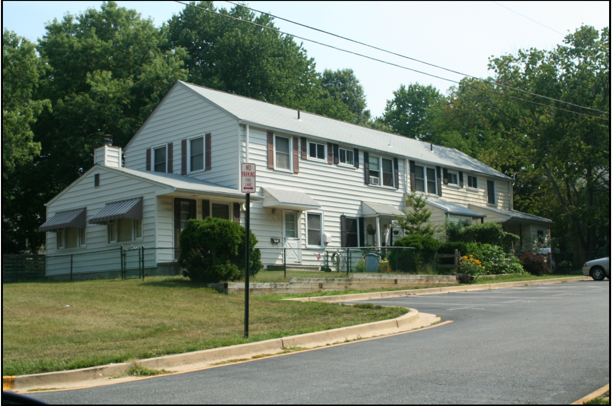
Looking northeast, 4 Laurel Hill Road ( EHT Traceries , 2007)
