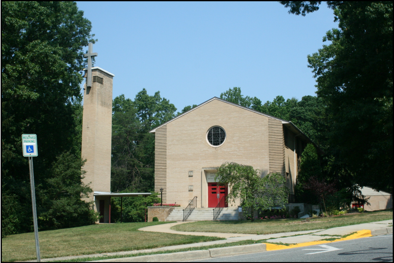
Looking west, 1 Hillside Road, Greenbelt Community Church ( EHT Traceries , 2007)
