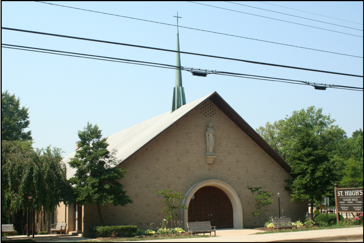
Looking south, 135 Crescent Road, St. Hugh's Catholic Church ( EHT Traceries, 2007 )
